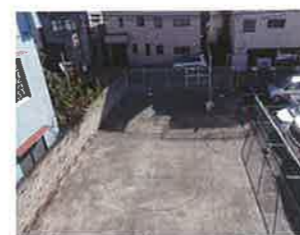
工事前の空き地 / Vacant ground before the start of construction
